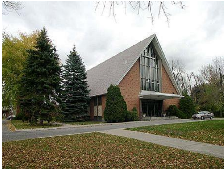
St.Francis of Assisi's Church
